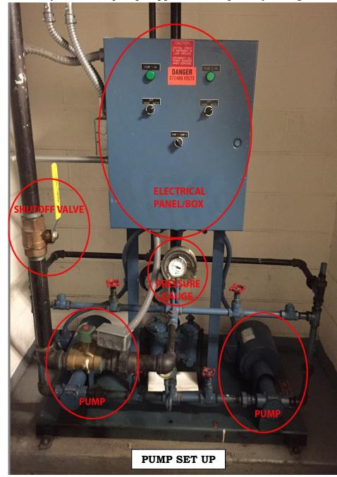
pumps will provide 100% of the maximum required flow. If the load is reduced, say in a burner, one pump may be adequate and the electrical demand will be reduced.
