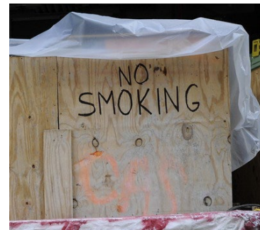
Unacceptable Warning Sign
