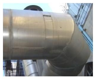
may cause carbon monoxide poisoning and burns. Warning signs shall be posted to instruct where it is dangerous and precautions must be taken. The integrity of the high temperature insulation around the exhaust ducts penetrating walls or roofs shall be verified periodically.
