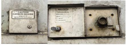
above any below-ground spaces or stairwells. There is no horizontal distance requirement. If installation of a fill connection is not practicable at particular premises, application shall be made for modification of the provisions of the Fire Rule before installing any carbon dioxide beverage dispensing system. Approval of such installation shall be subject to such additional safety requirements as the Department may require.
