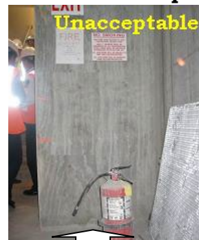
Improper floor placement of Fire Extinguisher.
