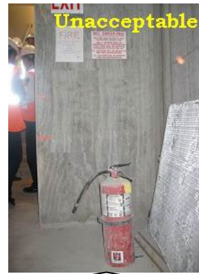
Improper floor placement of Fire Extinguisher.
