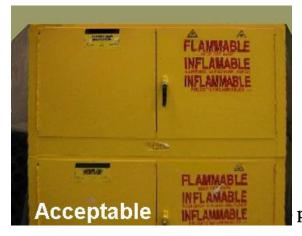
a conspicuous label in red letters on contrasting background which reads: FLAMMABLE-KEEP FIRE AWAY. The door must be well fitted, self-closing and equipped with a three-point latch. The bottom of the cabinet must be liquid-tight to a height of at least 2 inches.
