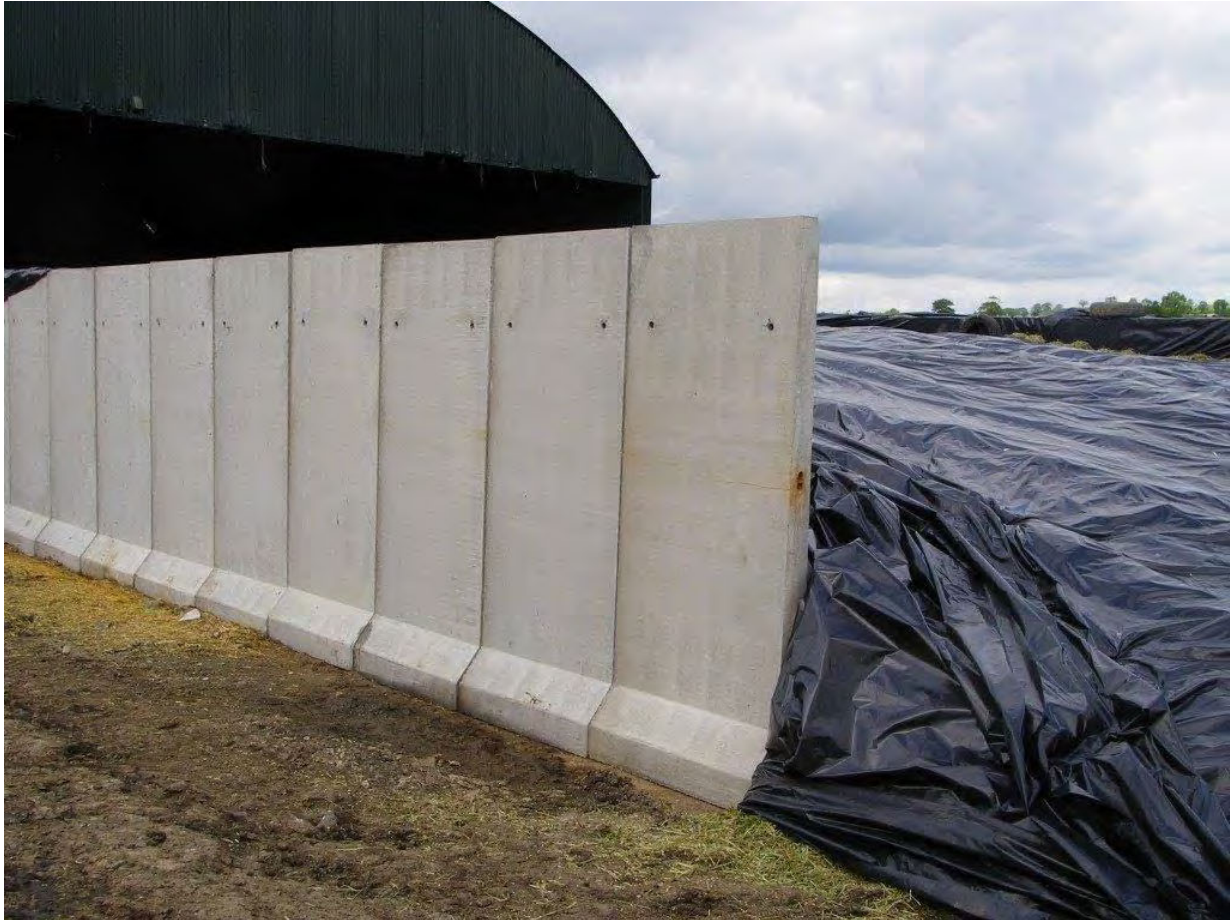
Precast concrete wall
