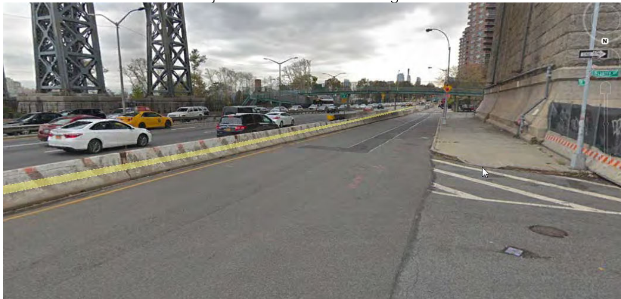
Street view of service road adjacent to Manhattan Bridge
