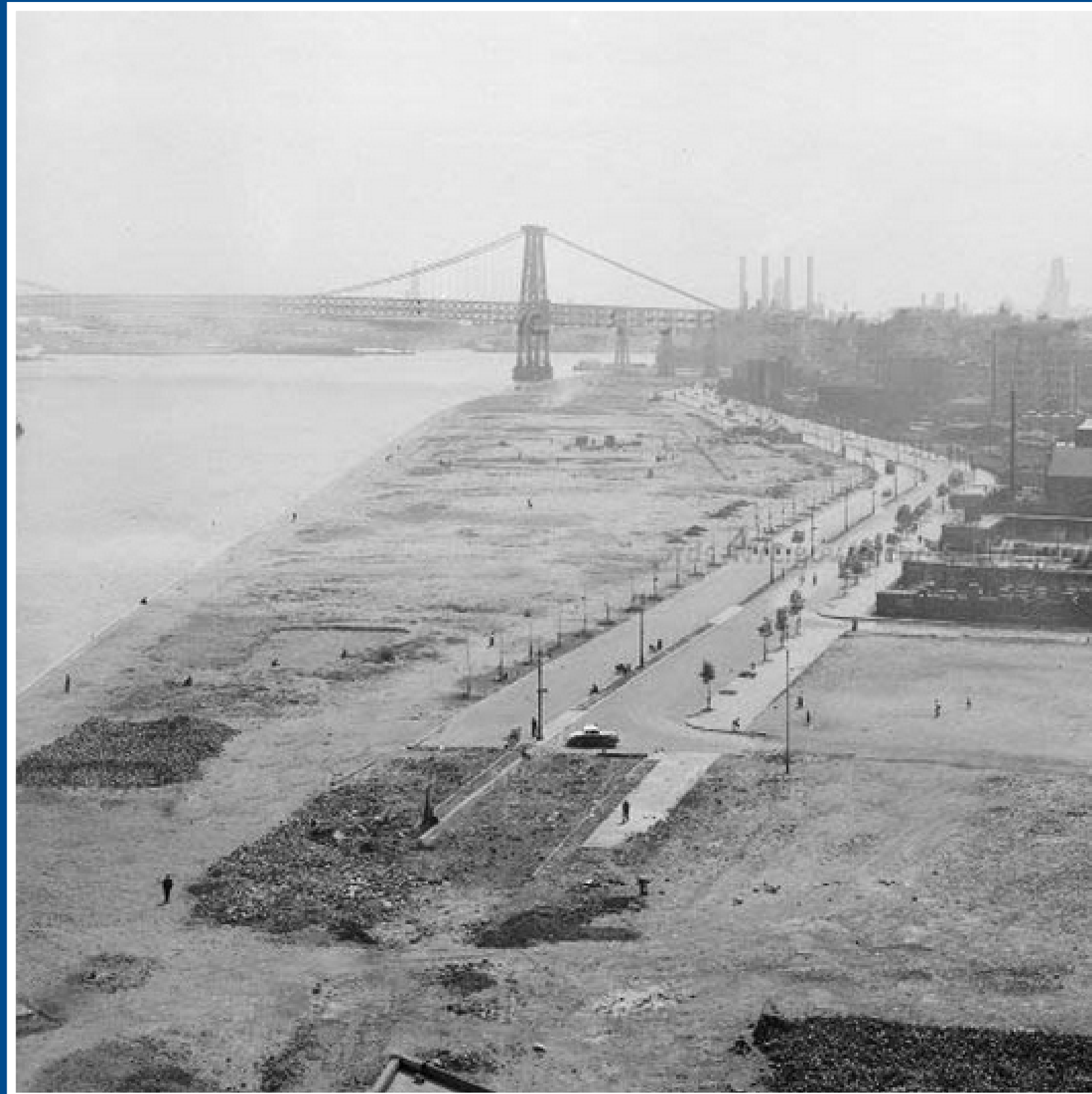
EAST RIVER PARK AND FDR UNDER CONSTRUCTION
