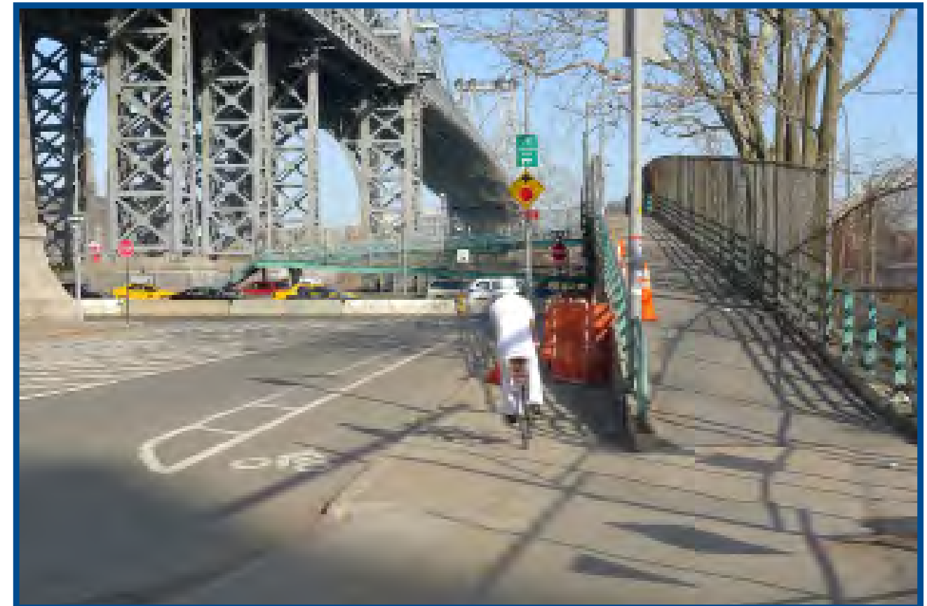
DELANCEY ST. BRIDGE ACCESS POINT
