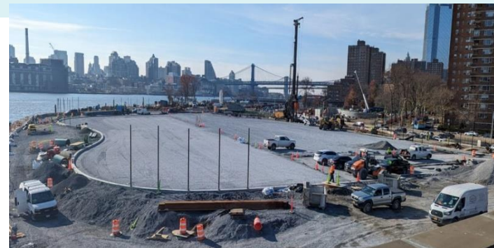
Ballfields 1 and 2 construction & lighting installation - November 2023
