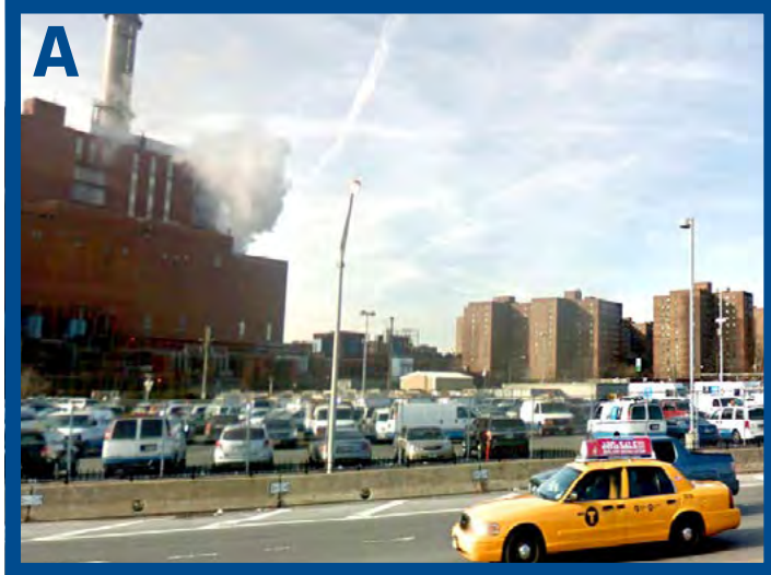
CON-ED PARKING LOT
