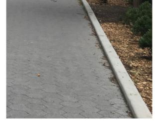
**STANDARD CONCRETE CURBS** 6" WIDE; FLUSH OR 2" HEIGHT POURED IN PLACE **AVERAGE CONCRETE**
