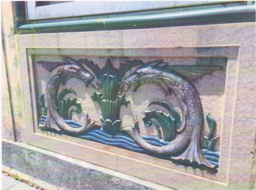
Photo 4: East River Park Track House Comfort Station river motif spandrel tile
