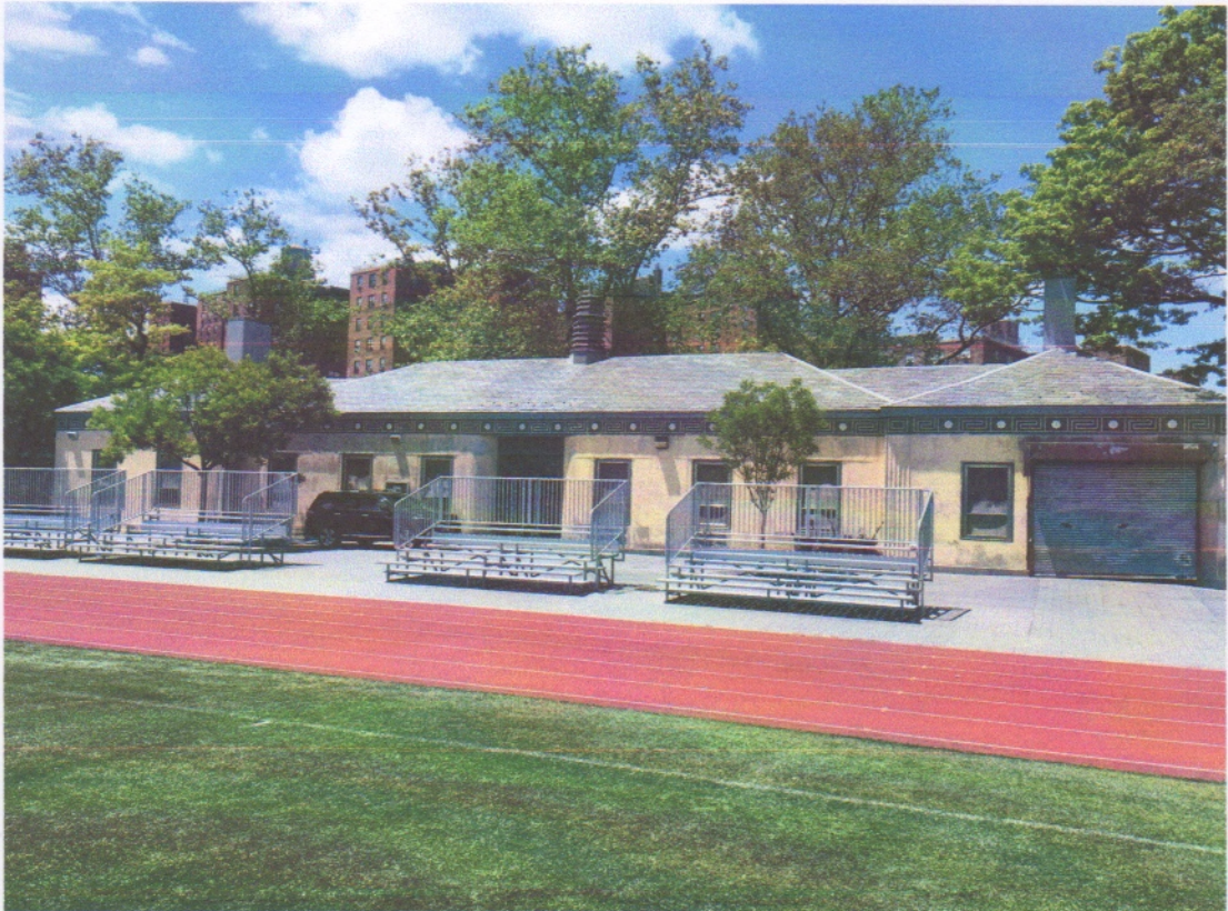
Photo 2: East River Park Track House Comfort Station
