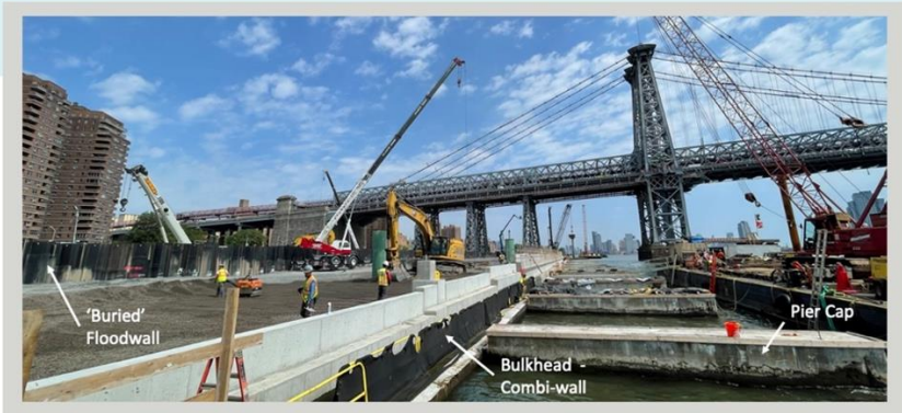
Future buried floodwall near Williamsburg Bridge, July 2023
