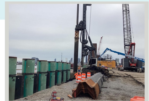
Combi-wall installation in East River Park, April 2023
