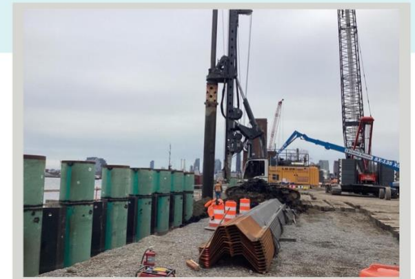
Combi-wall installation in East River Park, April 2023
