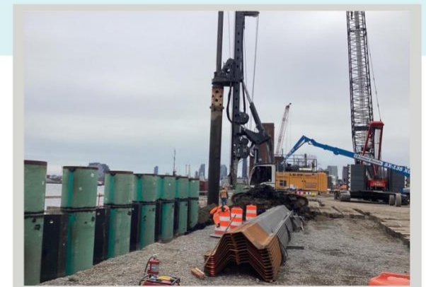
Combi-wall installation in East River Park, April 2023
