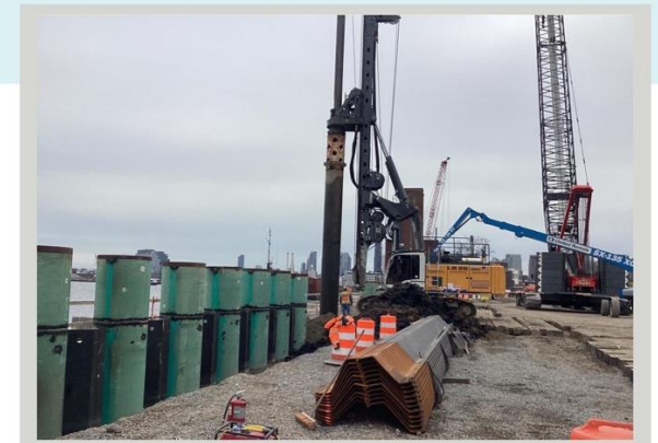
Combi-wall installation in East River Park, April 2023
