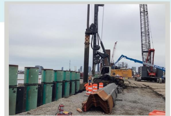
Combi-wall installation in East River Park, April 2023
