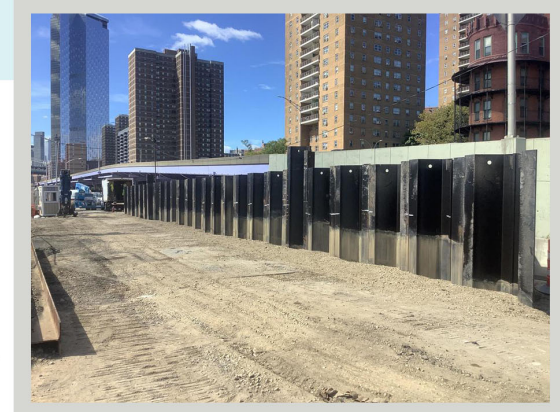
Sheet Pile for floodwall along the Greenway October 2022
