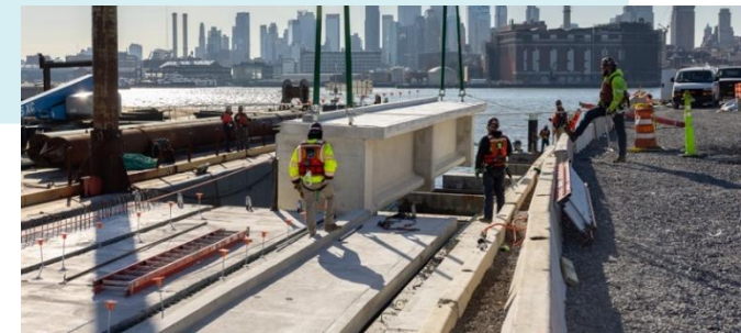
Pre-cast esplanade construction & installation - December 2023
