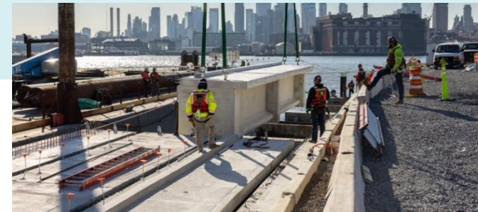
Pre-cast esplanade construction & installation - December 2023
