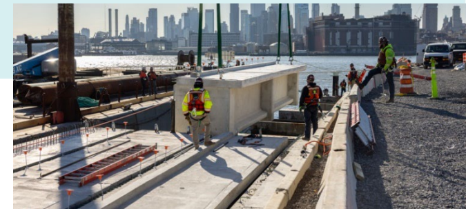
Pre-cast esplanade construction & installation - December 2023
