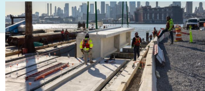
Pre-cast esplanade construction & installation - December 2023
