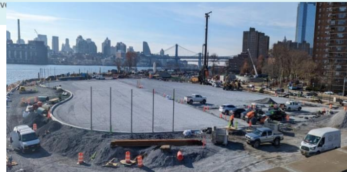
Ballfields 1 and 2 construction & lighting installation - November 2023
