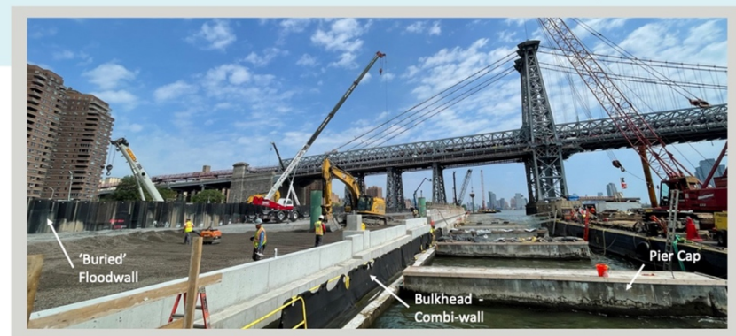
Future buried floodwall near Williamsburg Bridge, July 2023
