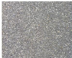
EXPOSED AGG. CONCRETE PAVEMENT W/ SAW CUT JOINTS PARK PATHWAYS
