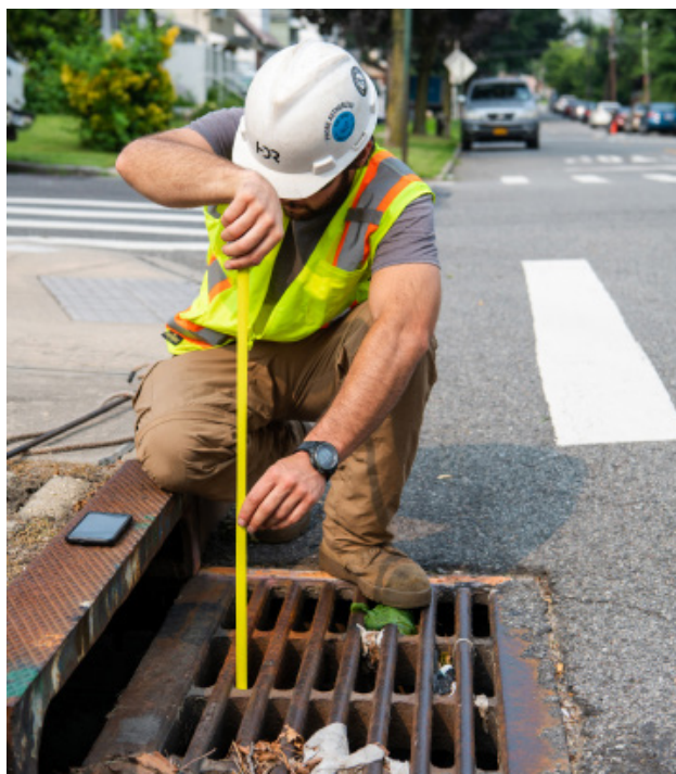
Measuring debris in catch basin for Loading Rate Study
