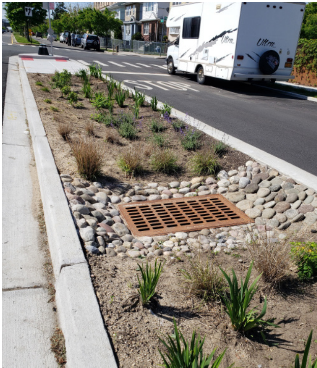
Rockaway Median Project
