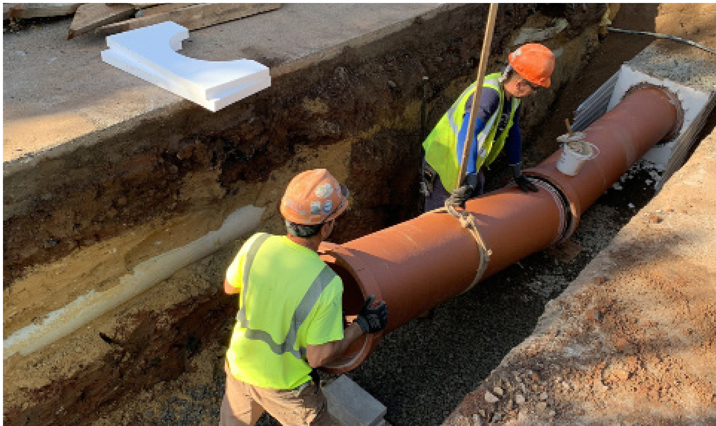
Installation of New Catch Basins for Willowbrook/Westerleigh
