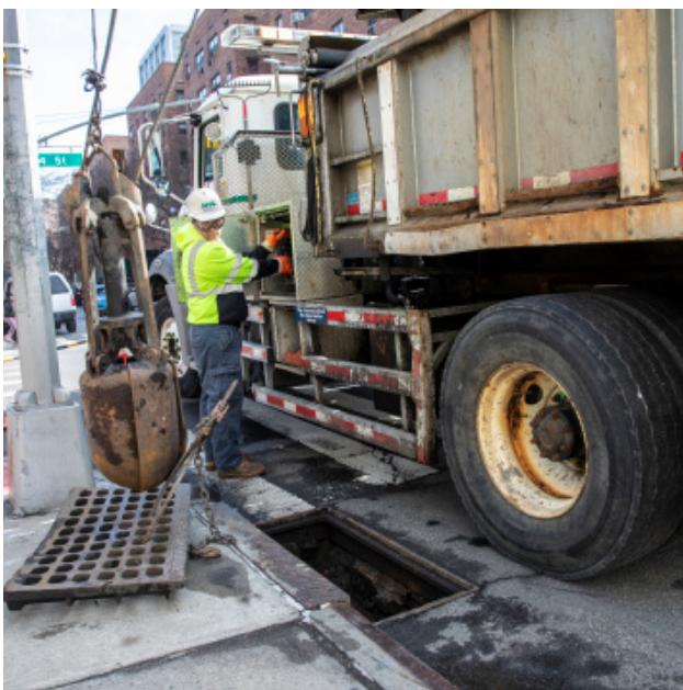
DEP catch basin cleaning
