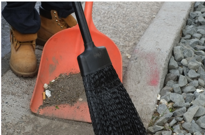
Remove sediment from curb cuts.
