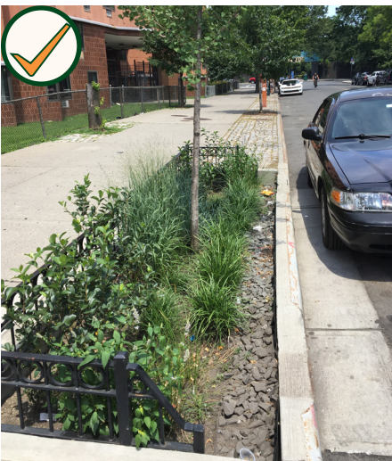
(Left) Shrubs and trees that have been trimmed stay within the rain garden. (Right) Overgrown plants can cause a tripping hazard.
