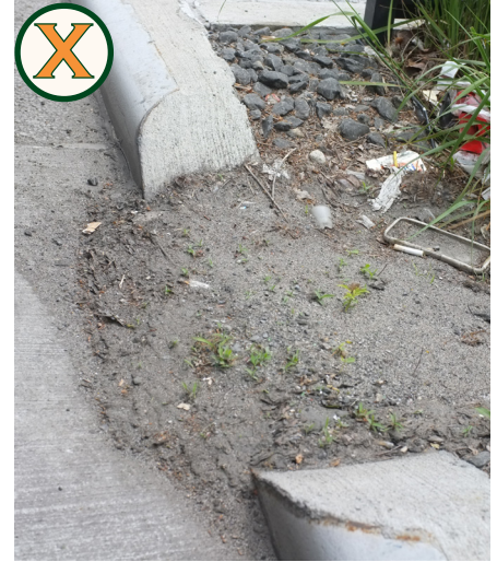
(Left) A clean curb opening for stormwater entering a rain garden. (Right) This curb cut is partially blocked with sediment and debris.
