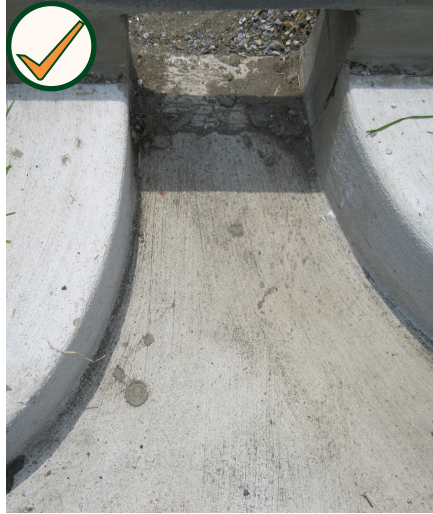
(Left) A clean curb opening for stormwater entering a rain garden. (Right) This curb cut is partially blocked with sediment and debris.
