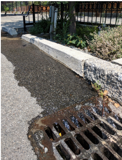
Stormwater flowing into a catch basin.
