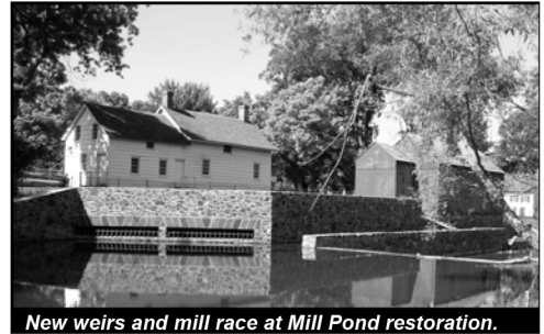
New weirs and mill race at Mill Pond restoration.
