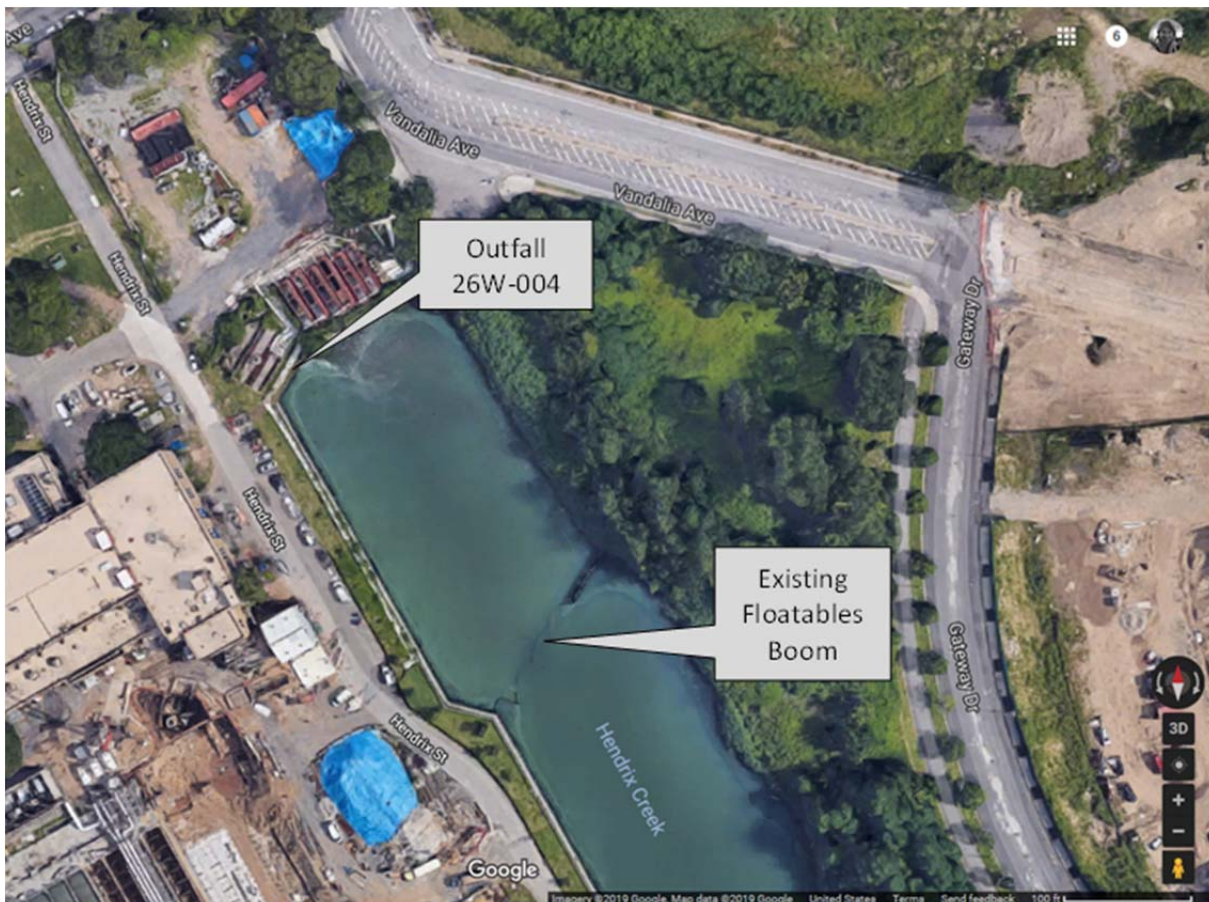
Figure 8-27. Location of Outfall 26W-004 and Existing Floatables Boom in Hendrix Creek
