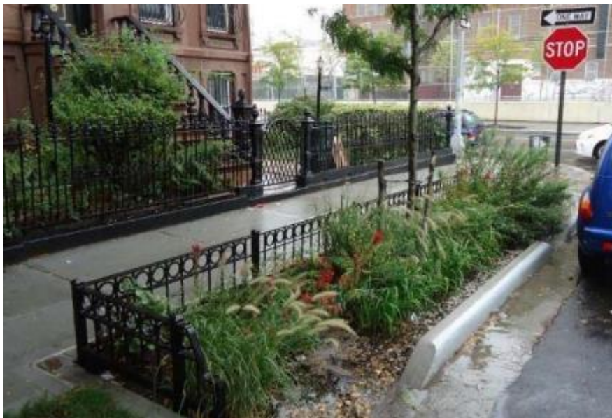
Figure 6-19: Example of a NYCDEP Rain Garden
