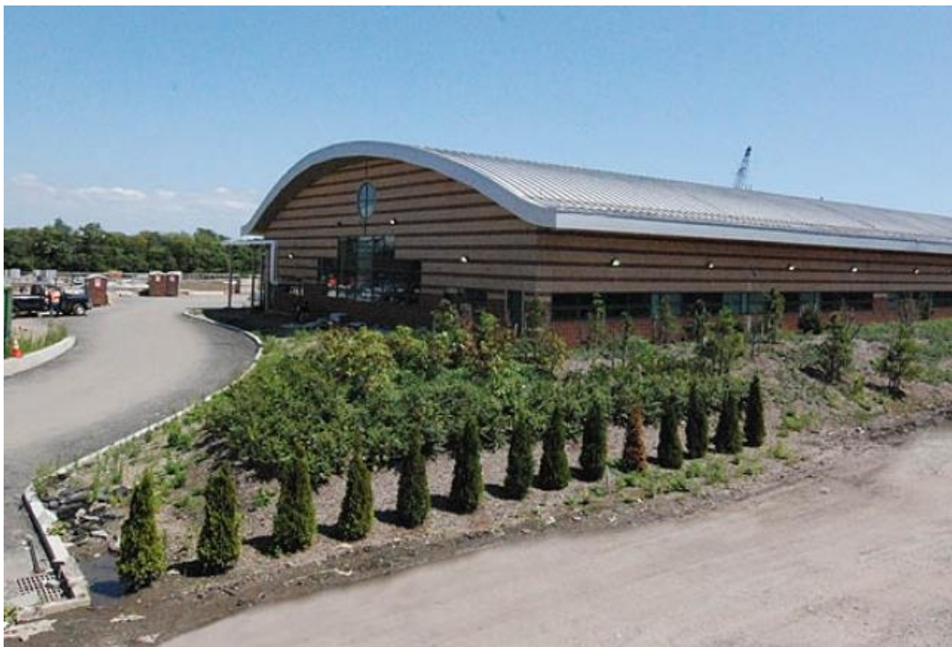
Figure 6-15: Paerdegat Basin CSO Retention Facility
