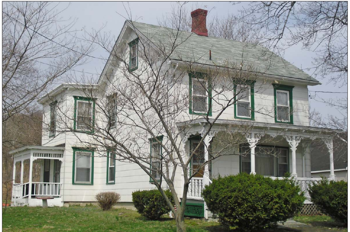
House at 5495 Route 9W 1a
