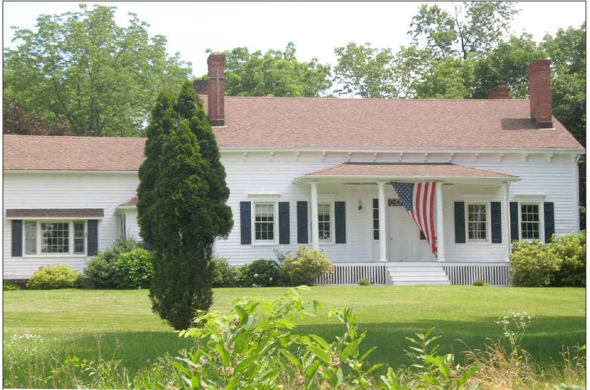
House at 225 River Road North, primary (south) facade 7
