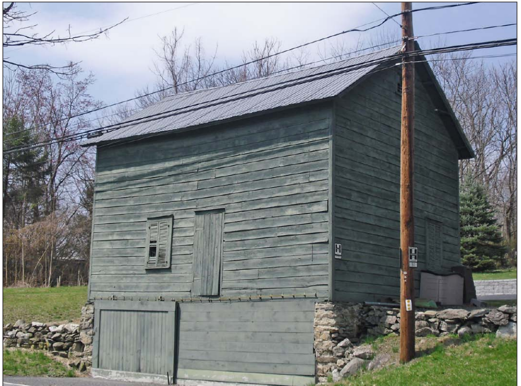
Barn at 51 Old Post Road 2b
