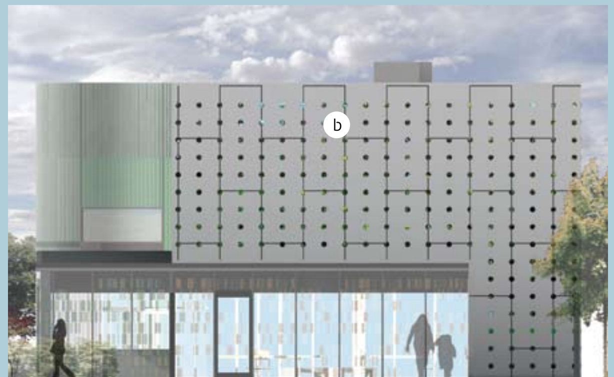
On the northern elevation of the library, the word Search is projected by sunlight through letter on the film of the parapet, illustration (a), above top, and onto the façade's glass curtain wall. The size and density of the letters
