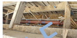
Installation of Sanitary Sewer on 119 th Ave.
