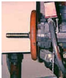
Stem out valve is OPEN
