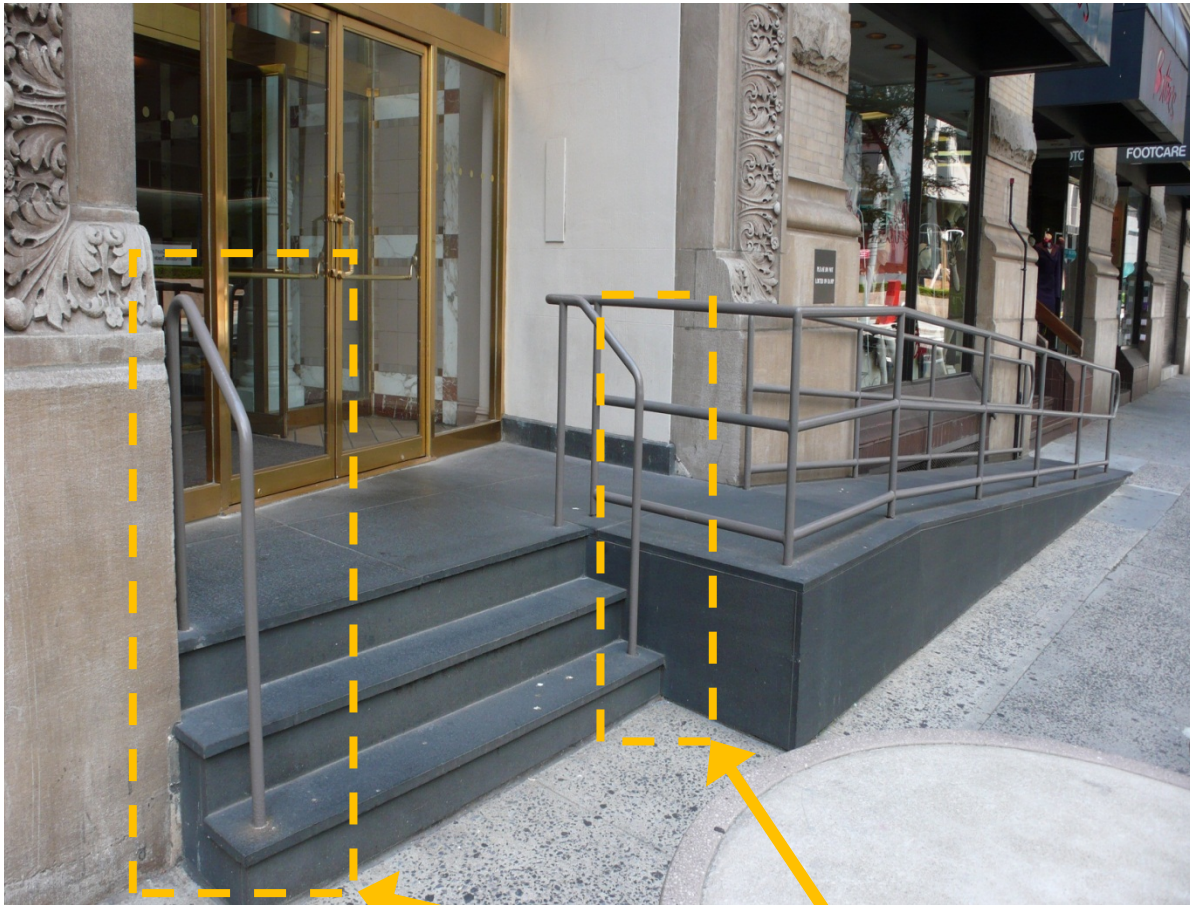
Fig. 505.10.2 Top Handrail Extensions at Stairs
