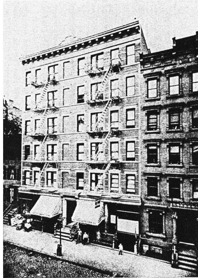
THE PROPER KIND OF TENEMENT HOUSE FIRE-ESCAPE — STAIRS.
