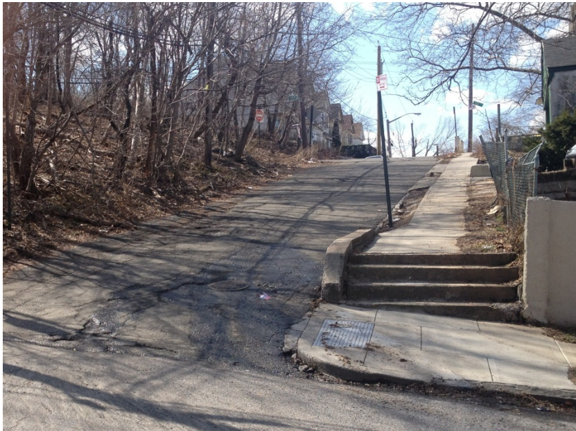
Hazards for persons with disabilities – provide Code compliant accessibility
