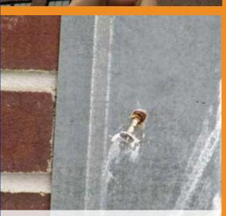
**FIGURE 10:** Close-up view of failed fasteners (Source: QEWI photo dated 2020. DOB archives)
