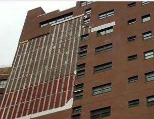
FIGURE 7: EIFS failure in mechanically attached EIFS (Source: DOB, 2020)
