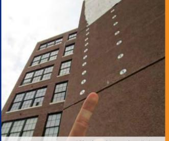
FIGURE 9: Emergency stabilization with post-installed anchors (Source: QEWI photo dated 2020. DOB archives)
