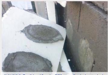
FIGURE 3: Traditional/barrier EIFS was adhesively attached to CMU substrate (Source: QEWI photo 2021. DOB archives)
