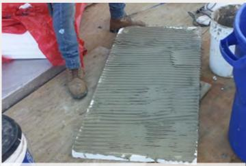
FIGURE 2: Barrier EIFS ready to be installed directly over a CMU substrate (Source: QEWI photo 2021. DOB archives)
