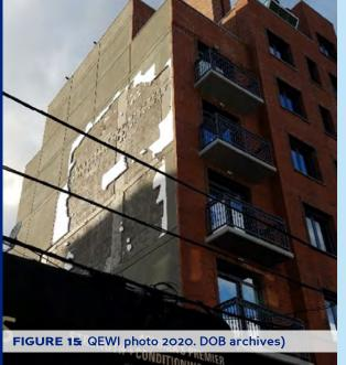
During a high wind event in August 2020, a 25'x25' area of EIFS cladding blew off the South façade of a recently constructed mixed-use building in Queens, falling on the roof of an adjacent building and on the sidewalk. In accordance with standard protocol for such incidents, the DOB ordered an engineering report of the 100% hands-on inspection of all the EIFS on the building.
