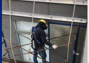
FIGURE 14: Reinforcement of the existing EIFS panels using brushed aluminum channels (Source: QEWI photo dated 2020. DOB archives)
