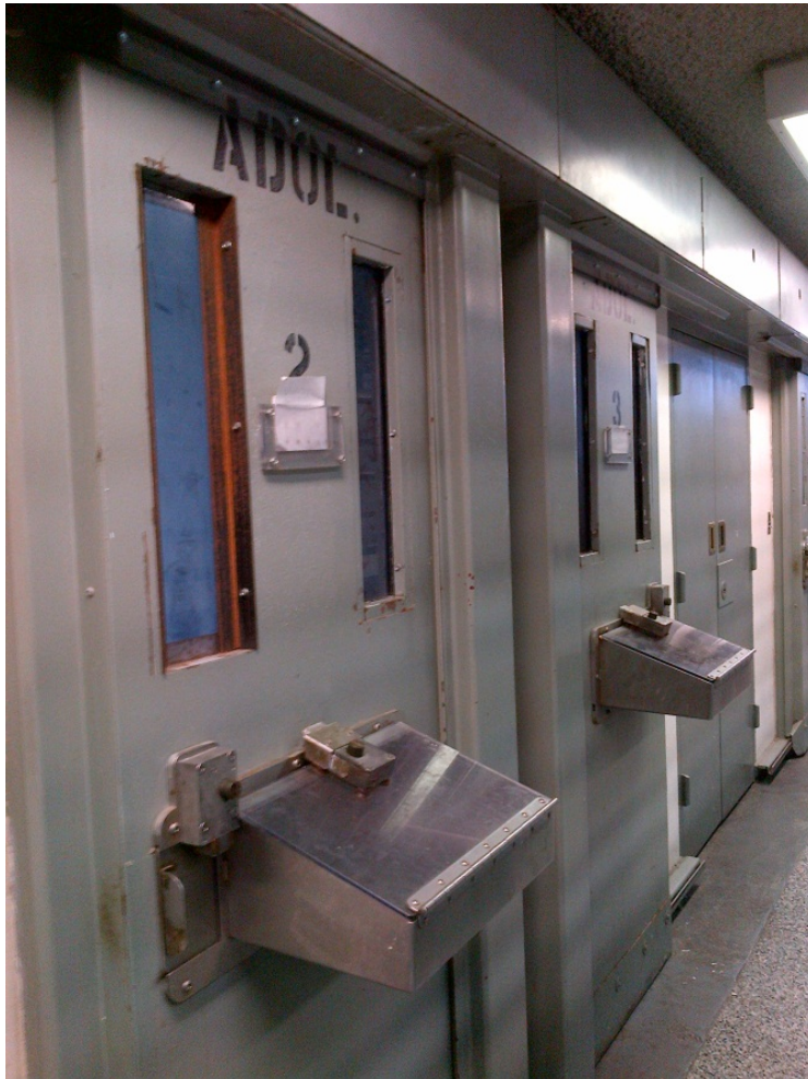
A view down one of the tiers in MHAUII. “ADOL” refers to adolescents. Each door has a “slot” through which food is delivered to prisoners. It also functions as a cuffing port, through which prisoners must place their hands for handcuffing before they exit their cell.
