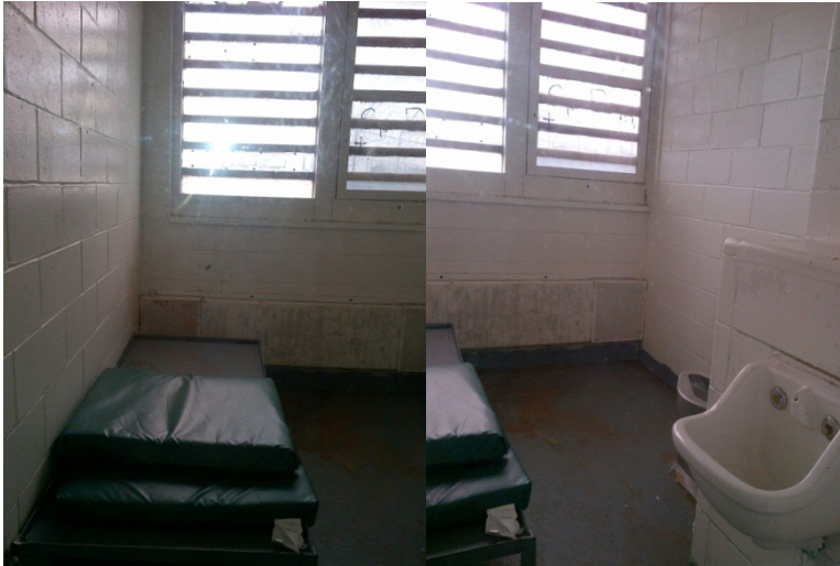
Two views of the interior of a vacant cell in punitive segregation
