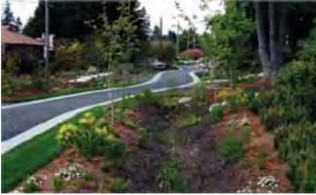
The vegetated swale adjacent to this path captures and infiltrates runoff.
