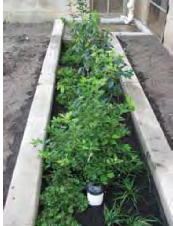
Runoff from this building is directed to a planter box to allow absorption by plants and soil, helping to reduce stormwater overflow events.
