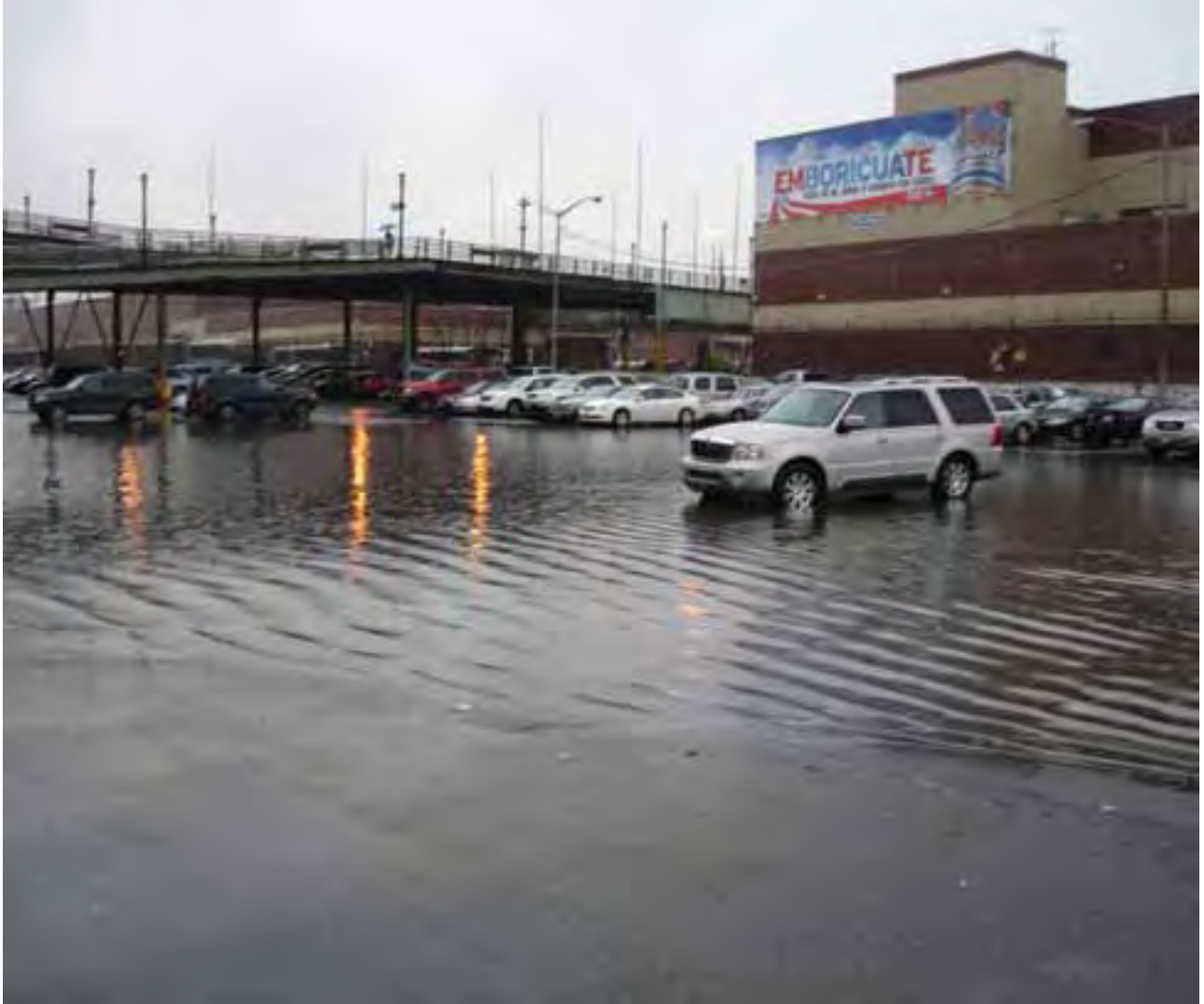
Heavy rains overload the city's stormwater system. Reducing pavement or using porous pavement in hardscapes such as parking lots will reduce the likelihood of flooding.
