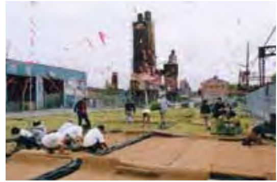
Spartina was raised in a constructed nursery onsite prior to planting along the shoreline. Netting above prevented birds from destroying the young seedlings.
