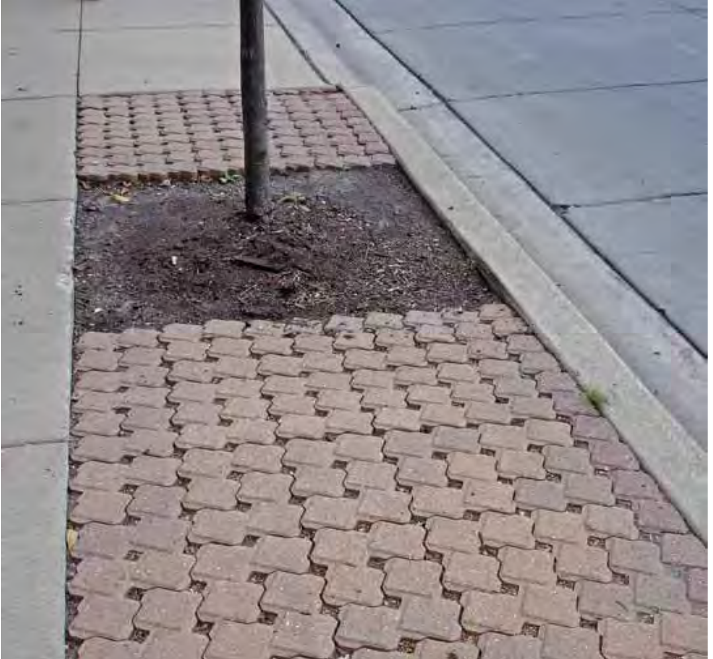
Porous paving over a portion of this tree pit allows for increased soil volume and infiltration without limiting pedestrian traffic.
