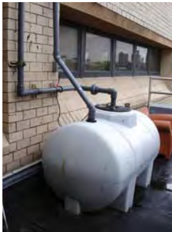
Rooftop runoff from the Parks' Maintenance Facility green roof on Randall's Island is directed to cisterns. The water captured by the cisterns is used to water the green roof during periods of drought.
