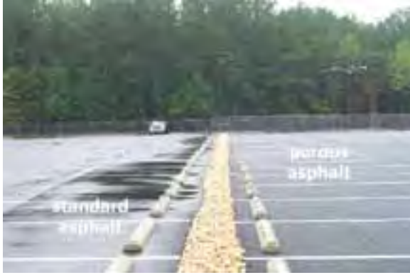
Stormwater runoff can pool on standard asphalt, as shown above. Porous asphalt allows water to drain directly through it, increasing ground water recharge and reducing icing in the winter.
