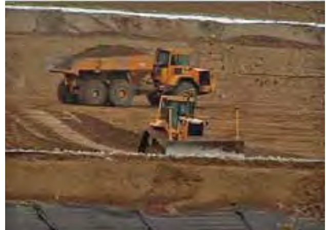
The Pennsylvania and Fountain Avenue landfills in Queens, operated as waste disposal sites in the 1950s and 60s, were capped with an impermeable membrane and covered by millions of tons of sand and topsoil brought in by barge. Analysis of regional soils and plant communities provided the blueprint for soil specifications on site.
