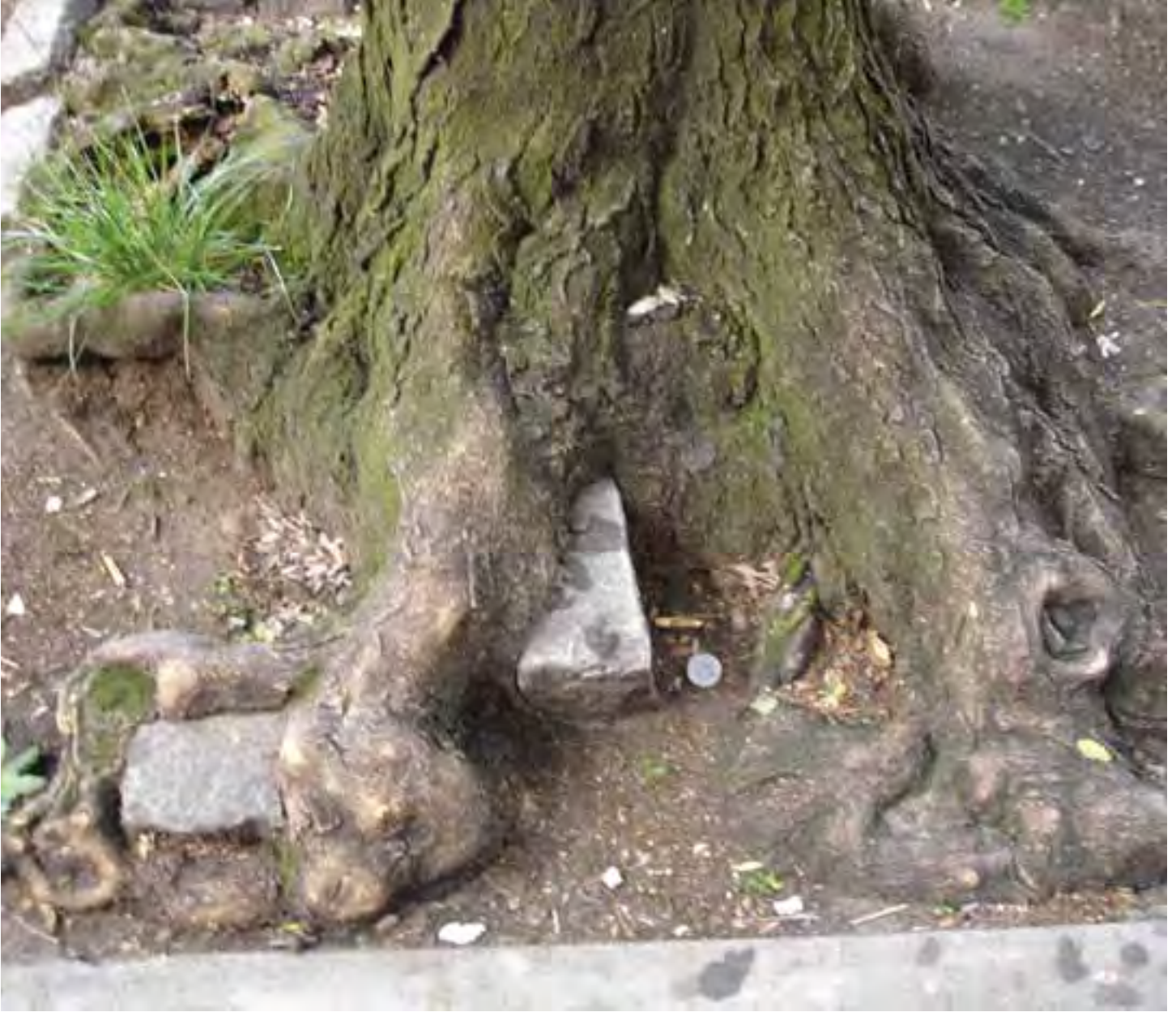
Street trees planted in adequate soil volumes are more likely to survive and cause fewer pavement breaks. This tree was not given enough soil, harming both the tree and the surrounding sidewalk.
