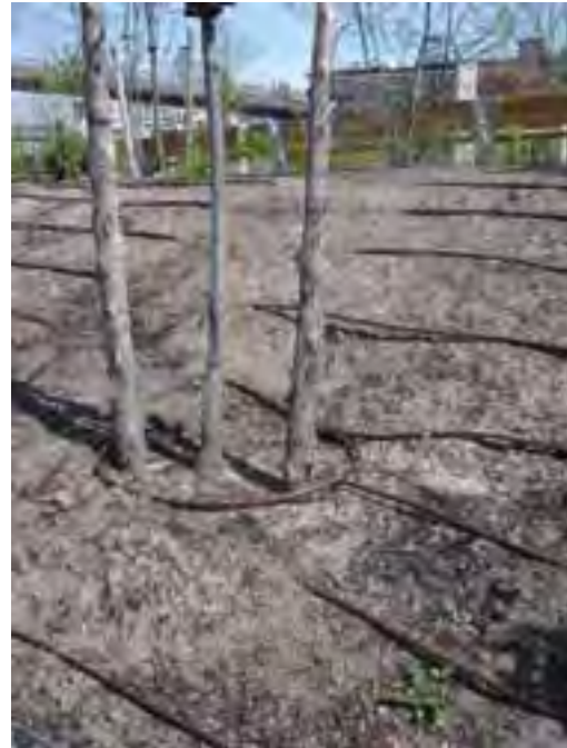
Engineered soil fiber amendments were added to the topsoil throughout Brooklyn Bridge Park to prevent erosion over the steep slopes. Also visible in this photo is the drip irrigation system, which was later covered with mulch.
