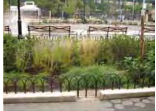
At Mullaly Park in the Bronx, breaks along the curb direct runoff into a planting bed whose engineered soil layers and water-tolerant plants are designed to retain water.
