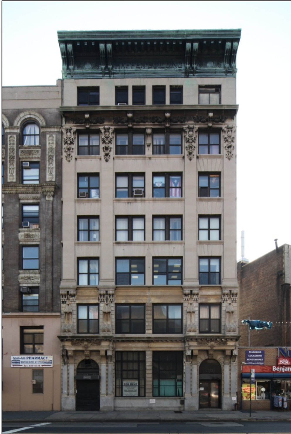
Haffen Building 2804-2808 Third Avenue (aka 507 Willis Avenue) Borough of the Bronx Tax Map Block 2307, Lot 59 Photo: Christopher D. Brazee, 2009
