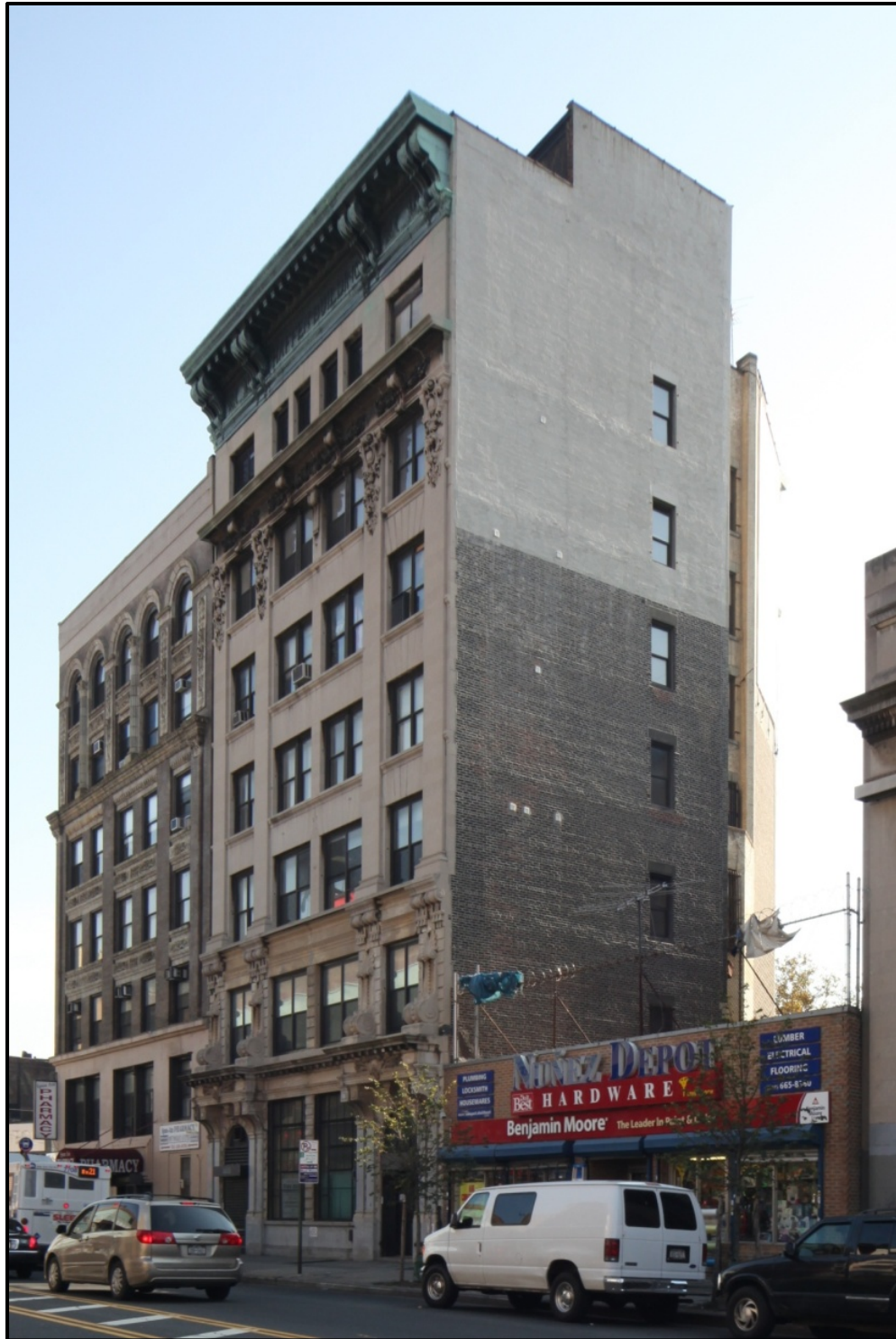
Haffen Building South Facade Photo: Christopher D. Brazee, 2009
