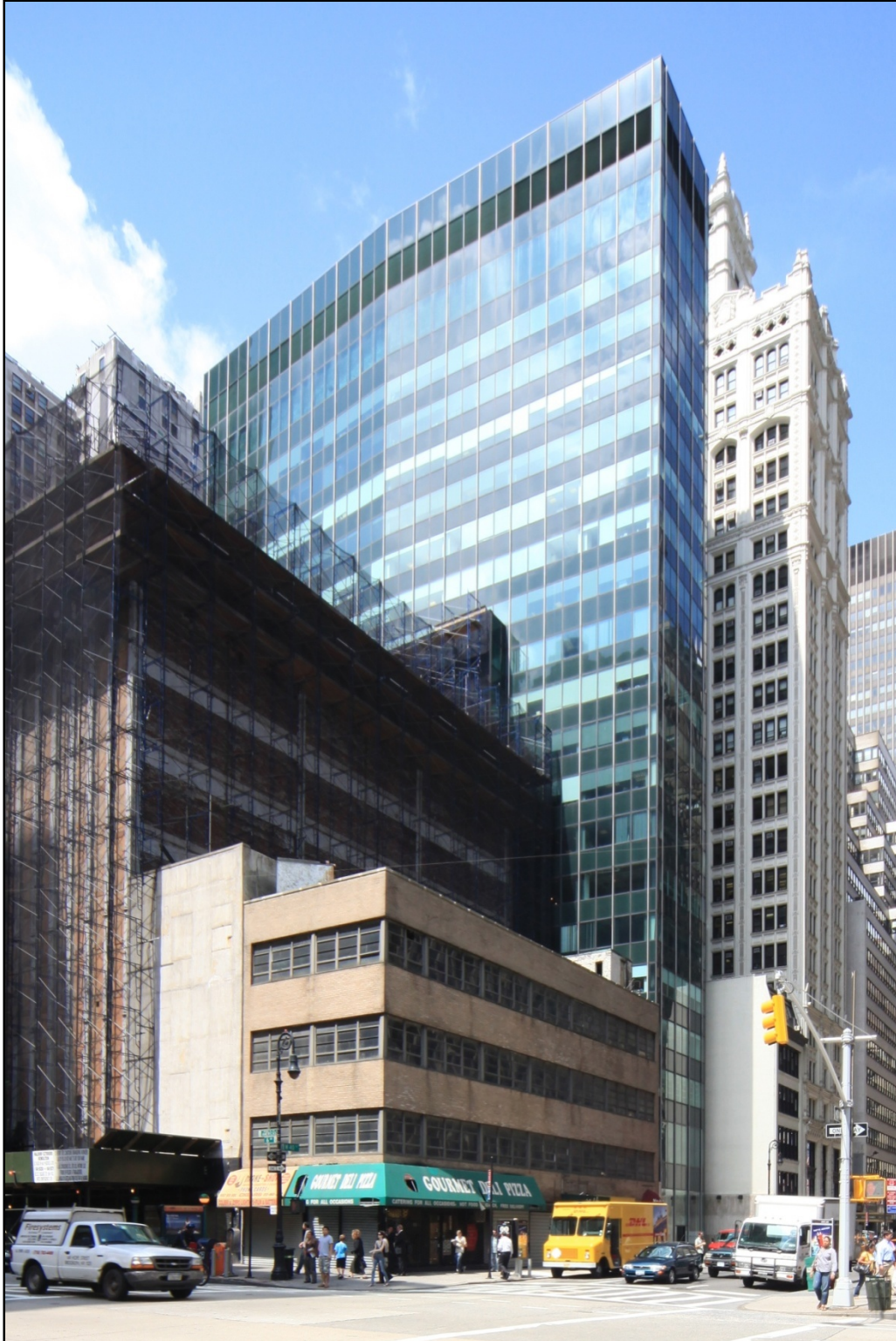
Springs Mills Building 104 West 40 th Street (aka 102-106 West 40 th Street, 107-15 West 39 th Street) Borough of Manhattan Block 815, Lot 21 East facade, view from Sixth Avenue Photo: Christopher D. Brazee, 2009
