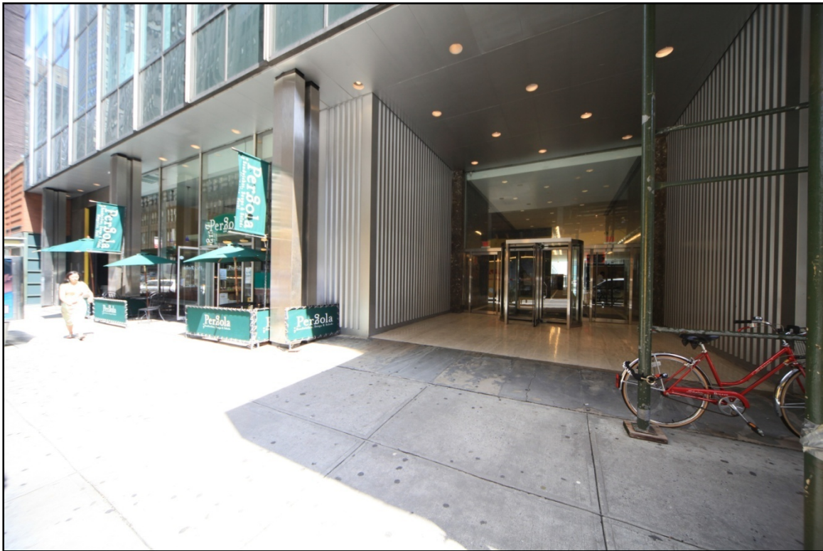
Springs Mills Building 39 th Street facade; first story arcade with breezeway Photos: Christopher D. Brazee, 2009
