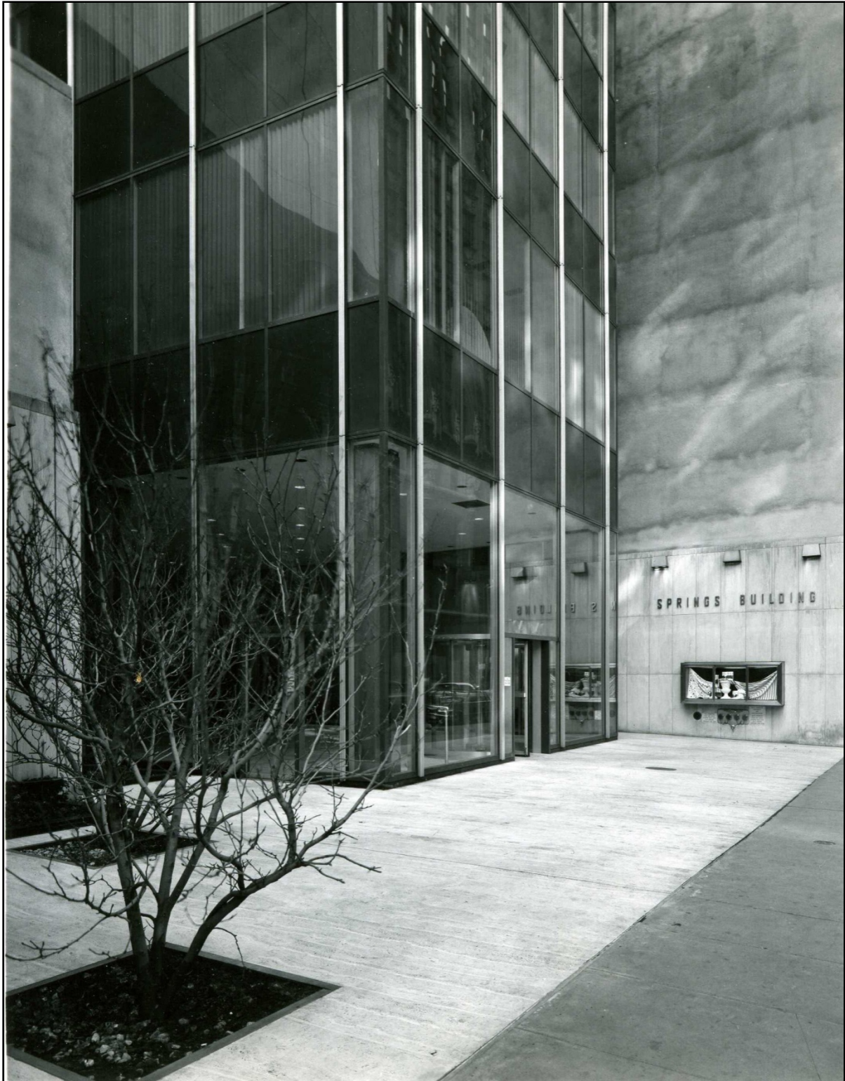
Springs Mills Building 40 th Street plaza Photo: Joseph W. Molitor, c.1963 Courtesy Abramovitz, Kingsland & Schiff
