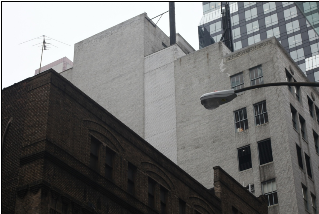
The Brill Building West 49th Street facade, lower floors, view toward Broadway Rear/west facade, upper floors, view from West 49th Street Photos: Christopher D. Brazee, 2009
