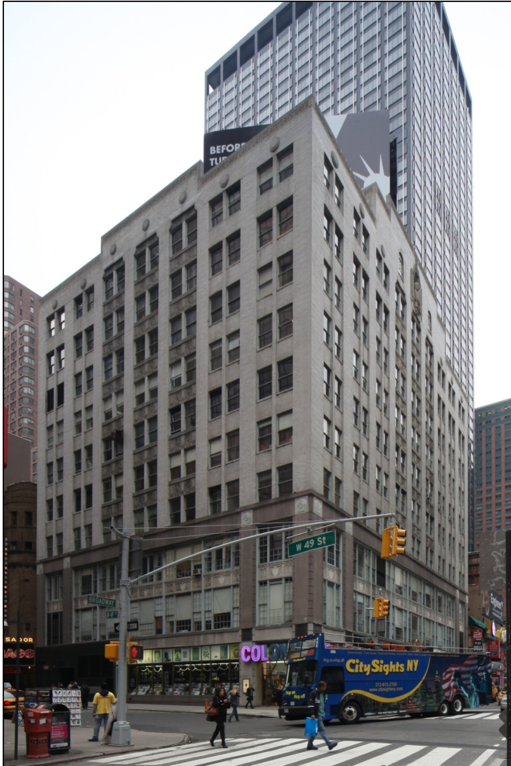
The Brill Building West 49 th Street and Broadway facades Photo: Christopher D. Brazee, 2009
