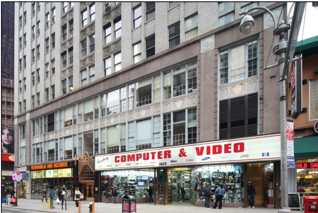
The Brill Building Broadway facade Window details and base Photos: Christopher D. Brazee, 2009
