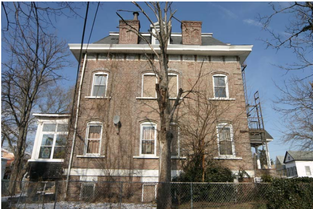
Schleicher House South façade, facing 123 rd Street, toward 14 th Avenue Photos: Christopher D. Brazee, 2009
