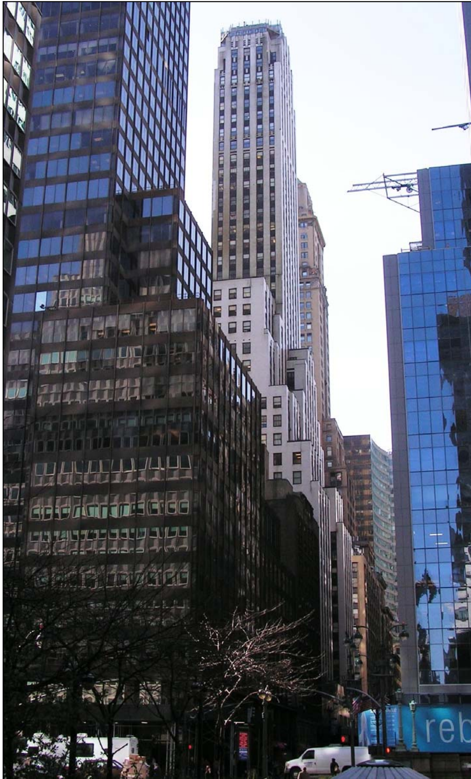
275 Madison Avenue East façade
