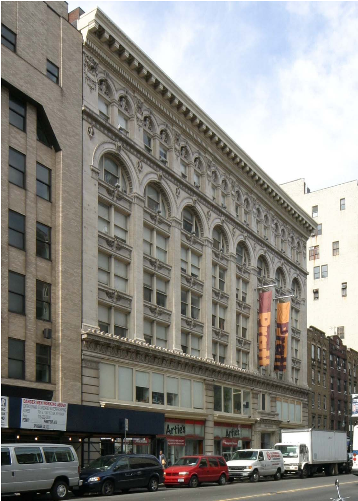
144 West 14 th Street (aka 136-146 West 14 th Street)
