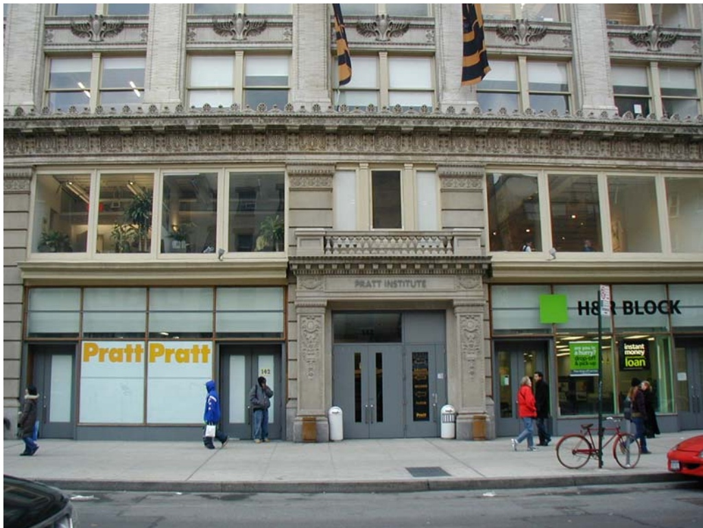
144 West 14 th Street Photos: Matthew A. Postal
