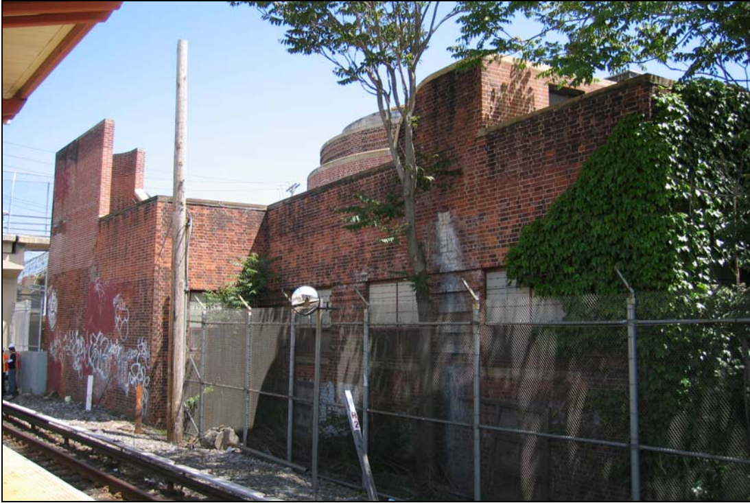
Tompkinsville (Joseph H. Lyons) Pool: North portion of west facade Photo: Tara Harrison, 2008
