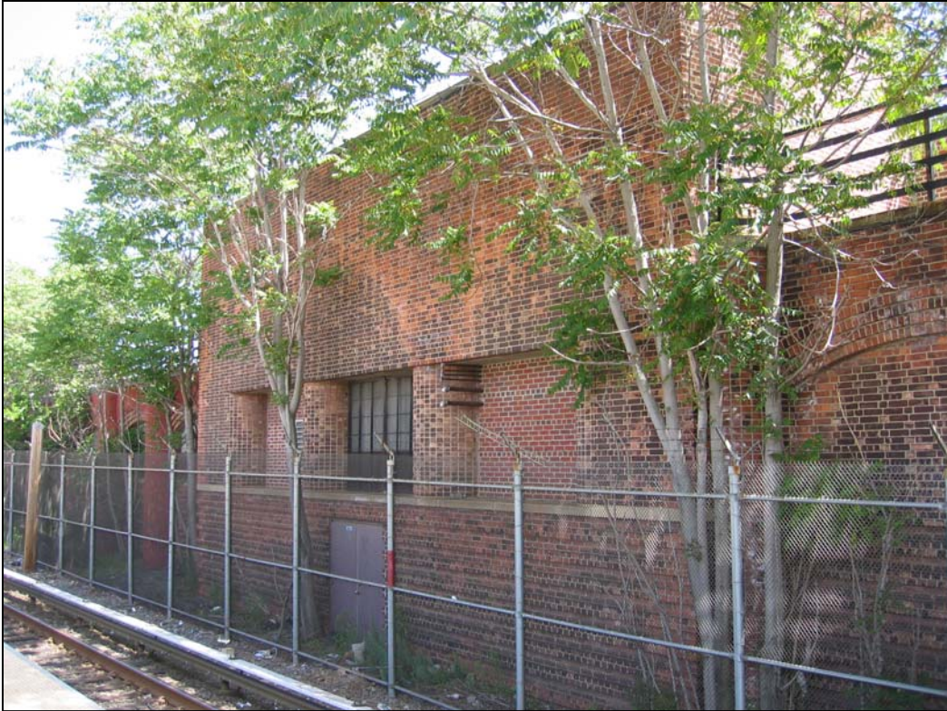
Tompkinsville (Joseph H. Lyons) Pool: Central portion of west facade Photo: Tara Harrison, 2008
