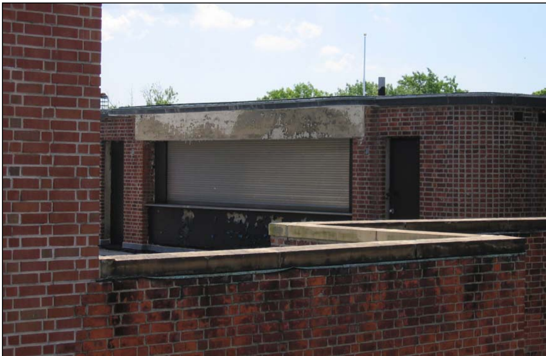
Tompkinsville (Joseph H. Lyons) Pool: Rooftop concessions stand Photo: Tara Harrison, 2008
