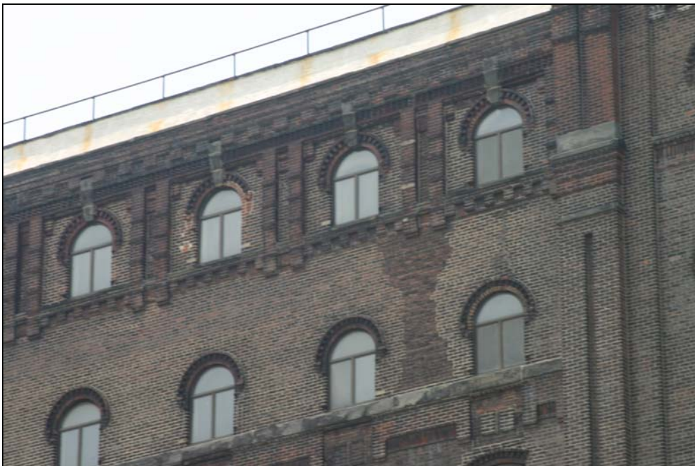
West facade, upper stories Photo: Carl Forster
